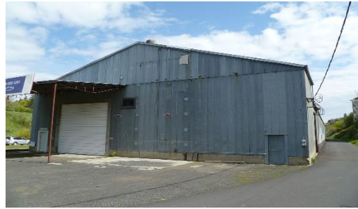
Horticultural products----- Storage facilities
